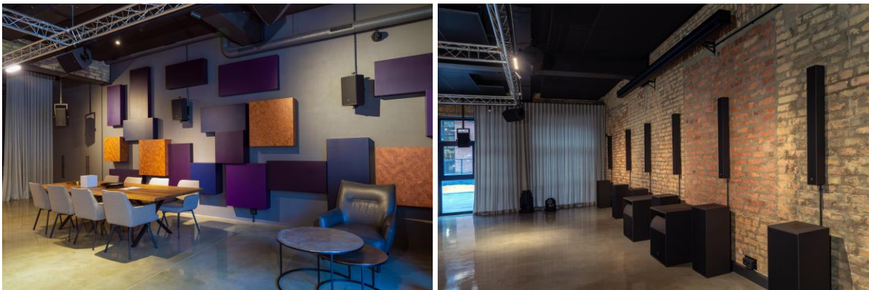
Figure 3. View on two opposite walls. To the left – wall membrane absorbers and furniture, to the right – L-ISA system loudspeakers.
